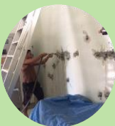
Pressure grouting & epoxy injection work
